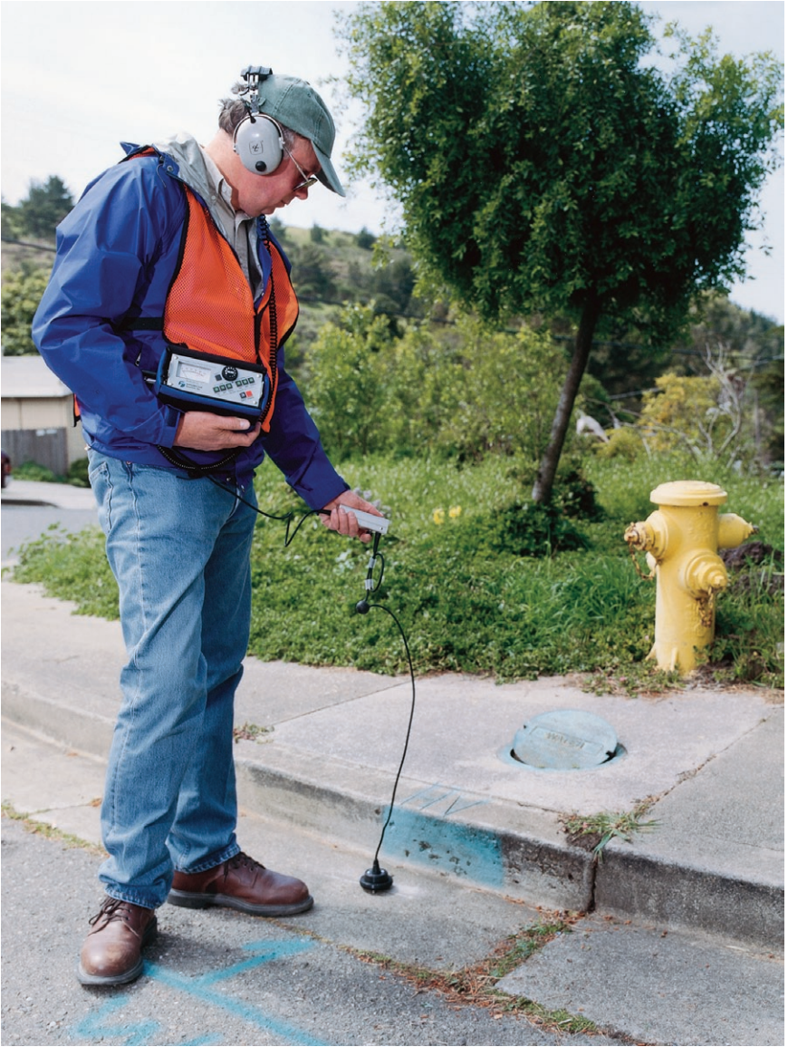
Figure 4-9 Leak Pinpointing Over a Hydrant Line
