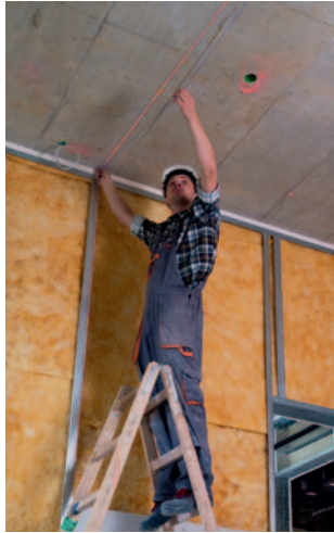
▲ Transfer of the layout from the floor to walls and ceilings.
