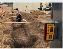
The Spectra Precision<sup>®</sup> CR700 Combination Laser Receiver is a machine mounted display receiver used on small grading and excavating equipment as well as a traditional laser receiver mounted to a grade rods. It is also ideally suited to work in vertical application for alignment control.
